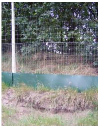
A spot on ecoduct Woeste Hoeve where wild boar dug for food. The fence still functions as a barrier because the wiring continuous below the surface level
